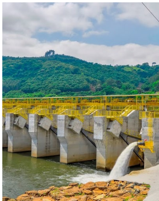
Image: Small Hydroelectric Power Plant Salto Goés, located in Tangara, Santa Catarina, Brazil. https://www.weg.net/institutional/US/en/solutions/energy
